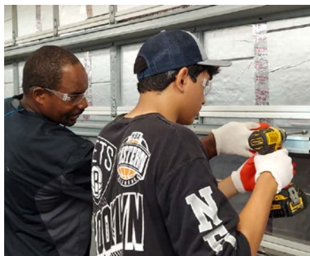
A TCBA boot camper learning from a Guaranteed Garage Repair technician.
